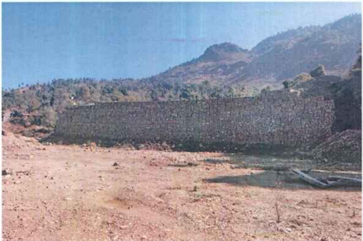
Gabion protection work at muck disposal site
