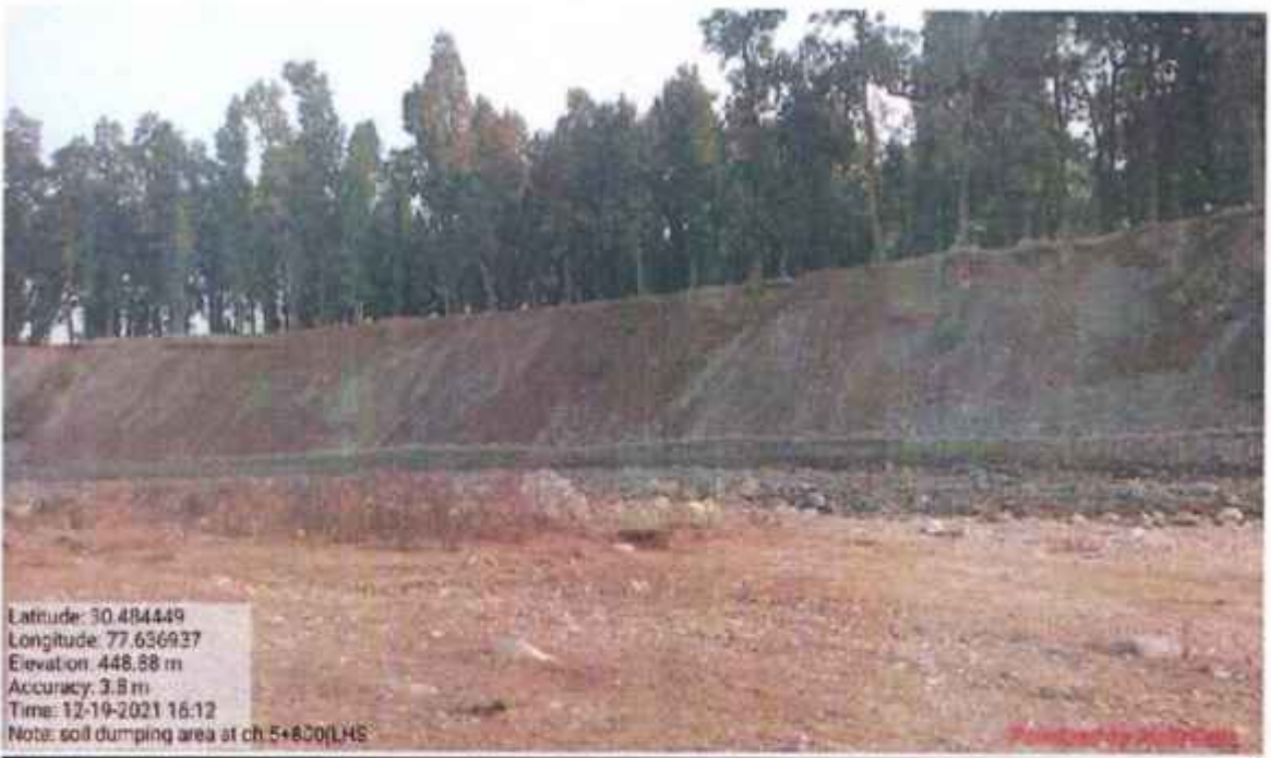
Gabion protection work at muck disposal site
