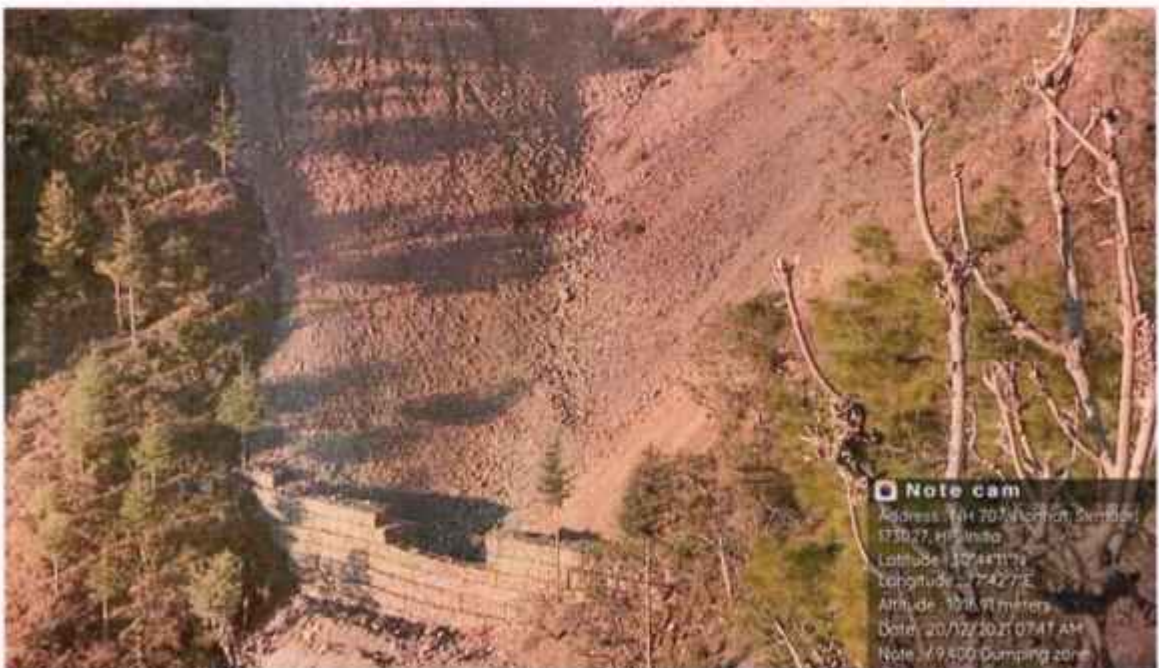
Gabion protection work at muck disposal site
