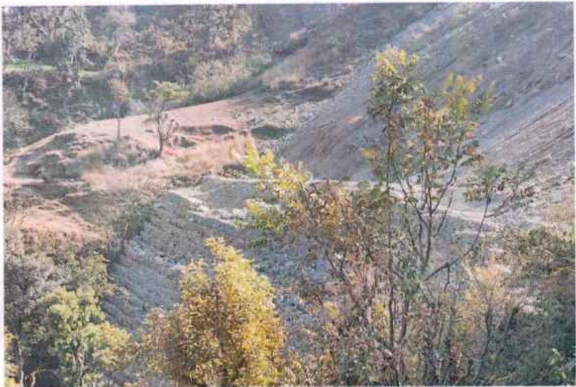
Gabion protection work at muck disposal site
