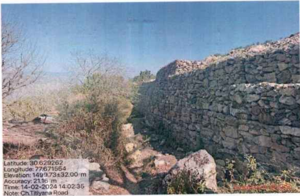
Gabion protection work at muck disposal site
