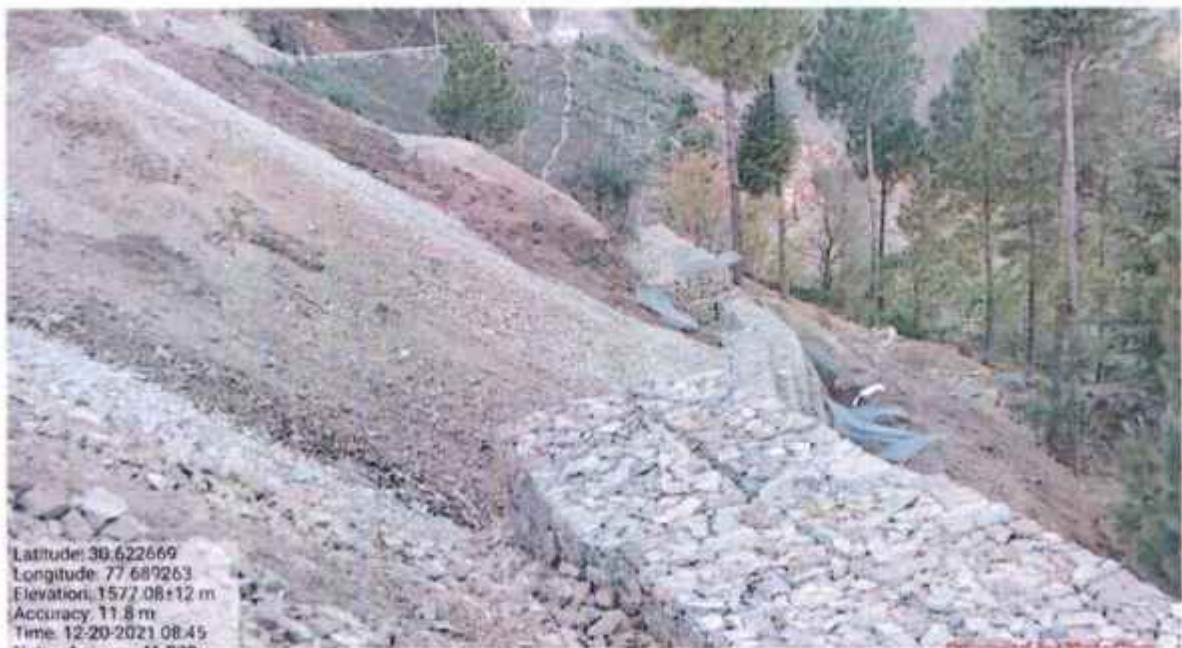
Gabion protection work at muck disposal site
