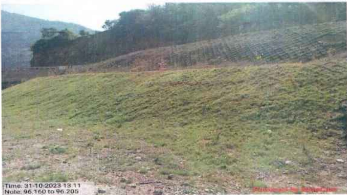
Geocell with hydroseeding and bamboo plantation
