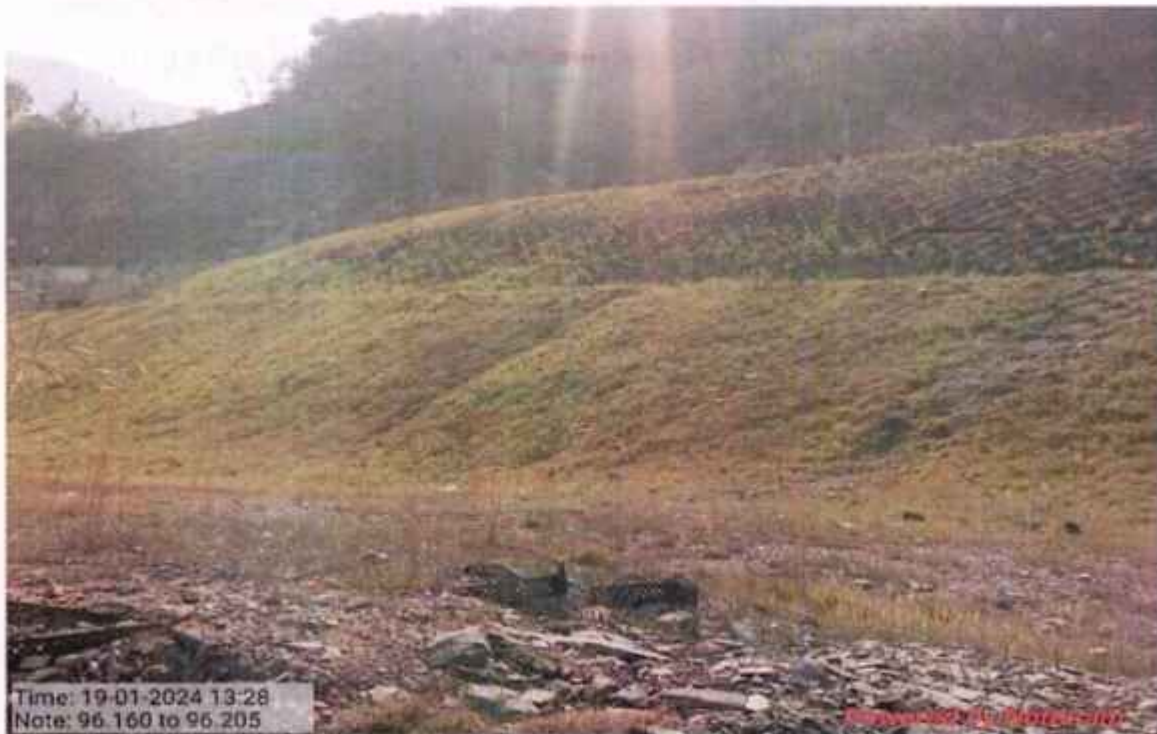
Geocell with hydroseeding and bamboo plantation
