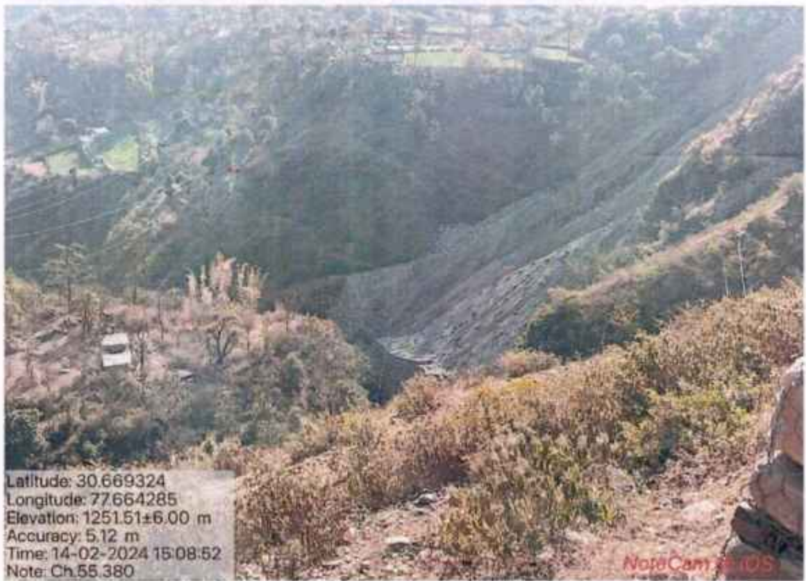
Gabion protection work at muck disposal site
