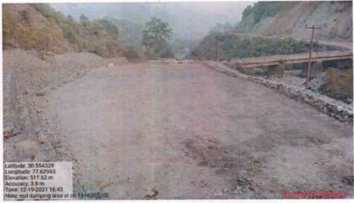
Development of park and gabion protection work at muck disposal site
