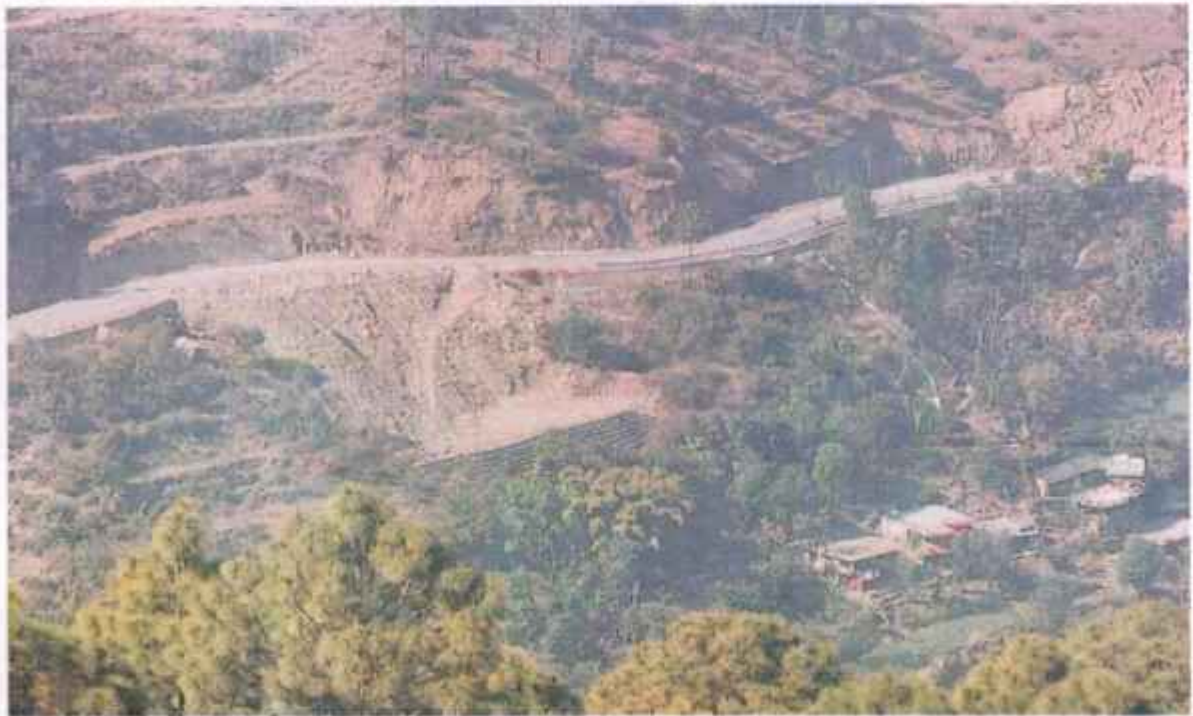
Gabion protection work at muck disposal site
