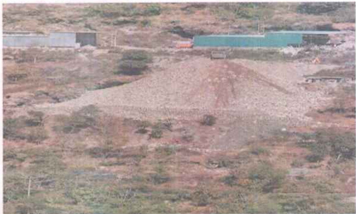
Gabion protection work at muck disposal site
