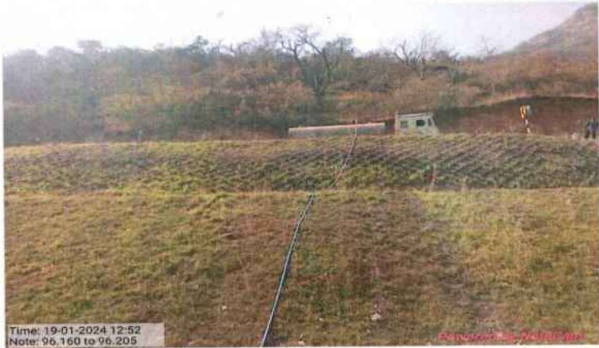
Geocell with hydroseeding and bamboo plantation
