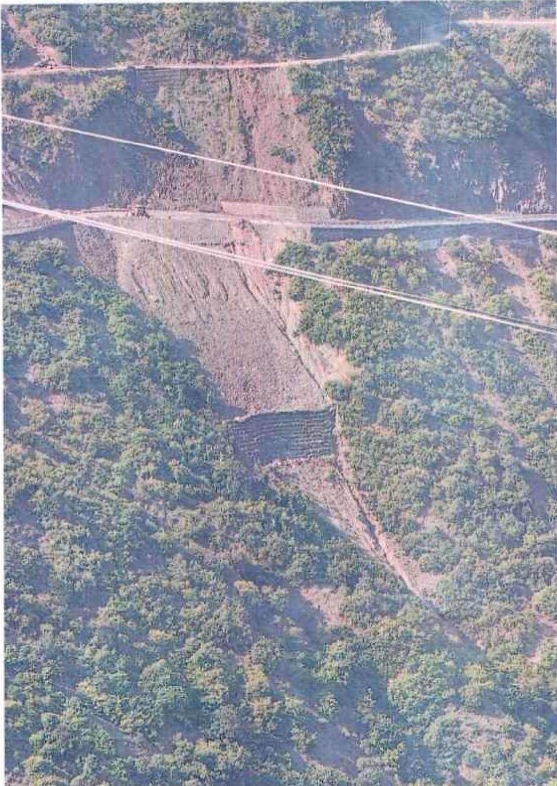
Gabion protection work at muck disposal site
