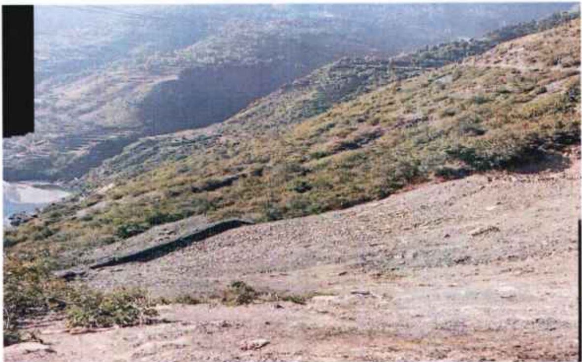
Gabion protection work at muck disposal site
