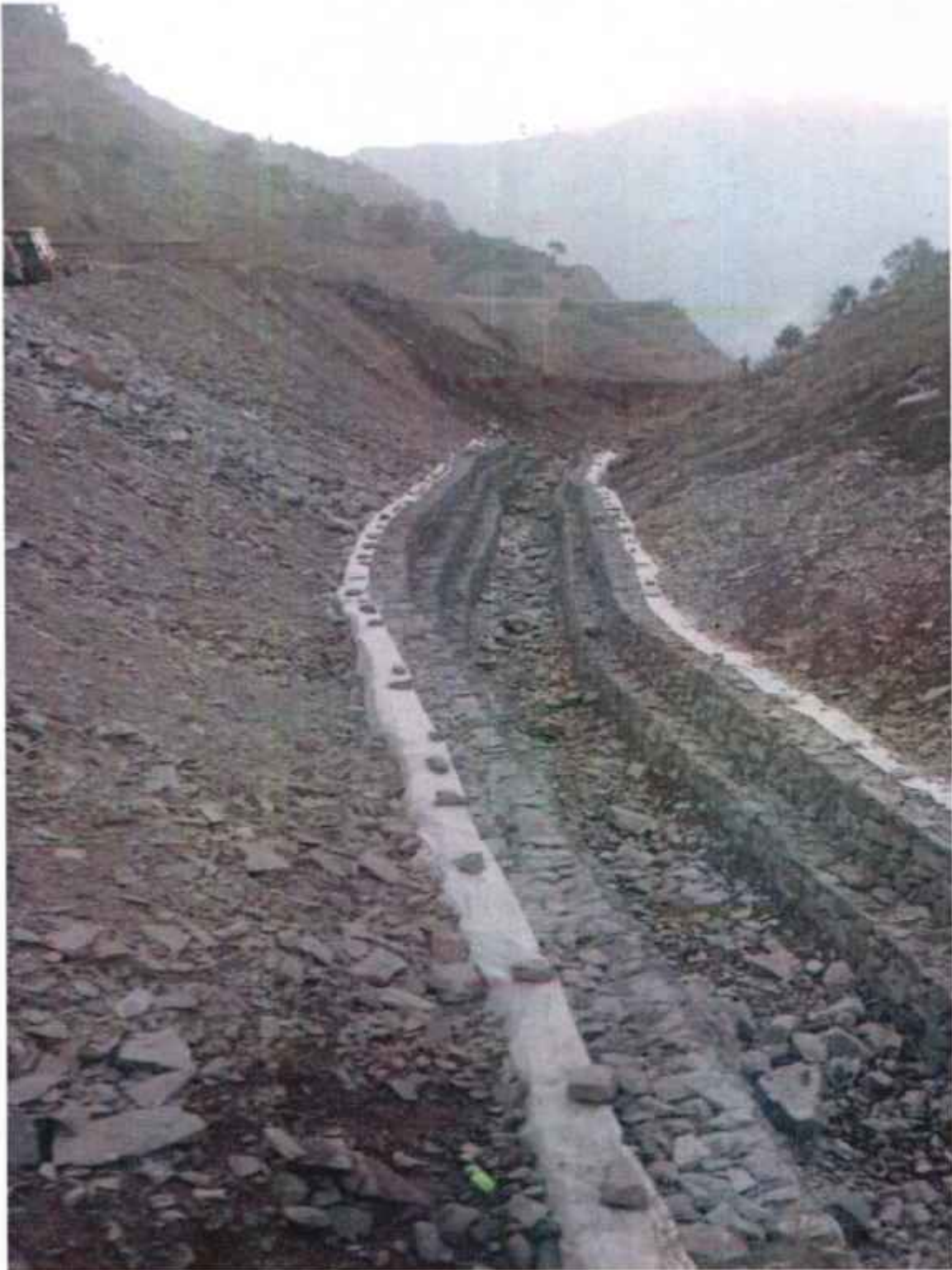
Water channelization work at muck disposal site
