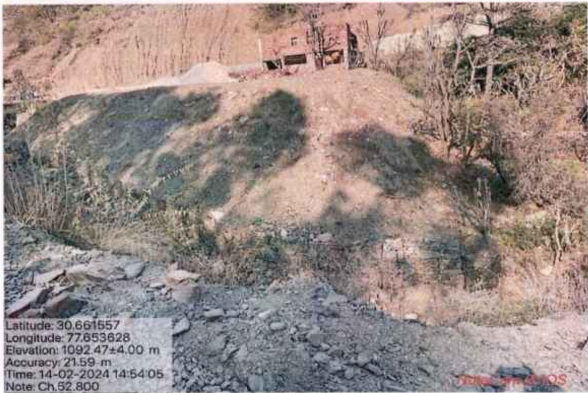
Gabion protection work at muck disposal site
