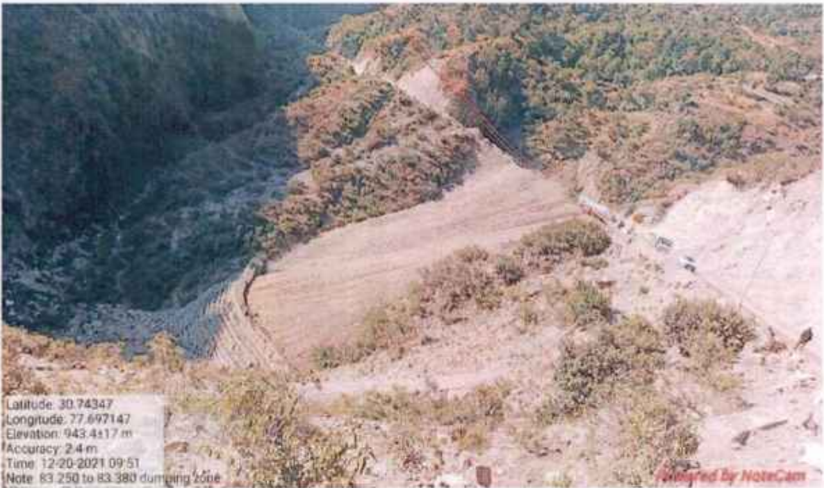
Gabion protection work at muck disposal site
