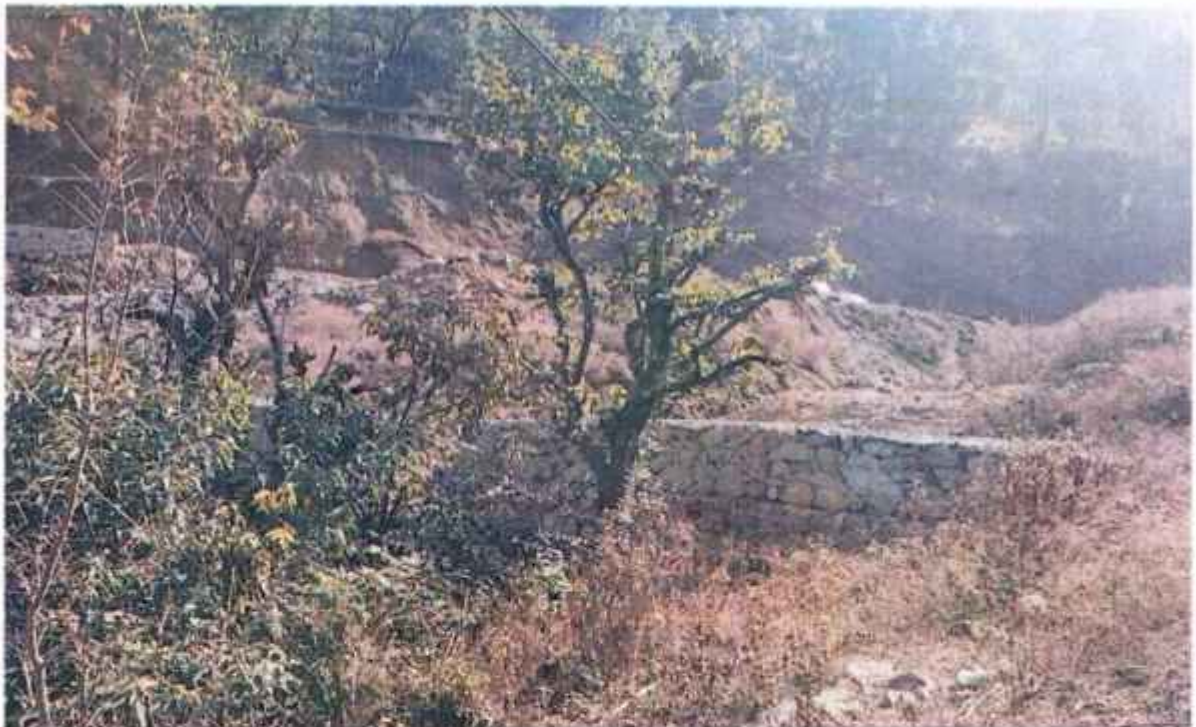
Gabion protection work at muck disposal site
