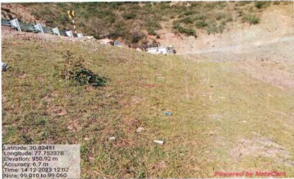
Geocell with hydroseeding and bamboo plantation
