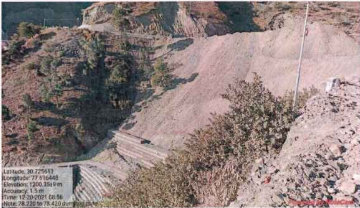
Gabion protection work at muck disposal site
