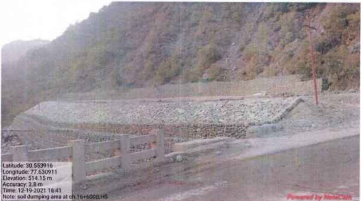
Development of park and gabion protection work at muck disposal site
